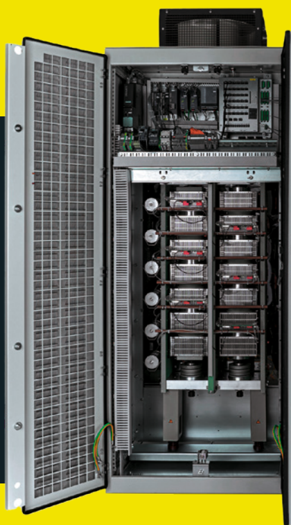
Single 6-pulse rectifier
