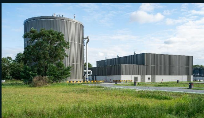
ENECO wastewater treatment facility in Utrecht
