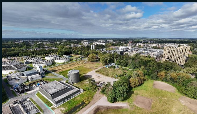
ENECO wastewater treatment facility in Utrecht
