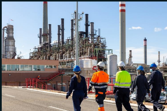
Repsol's Puertollano Olefins Plant in Spain
