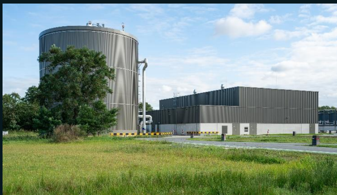
ENECO wastewater treatment facility in Utrecht
