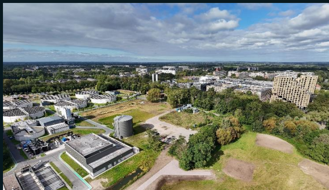
ENECO wastewater treatment facility in Utrecht
