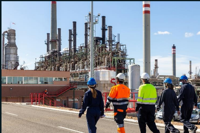
Repsol's Puertollano Olefins Plant in Spain
